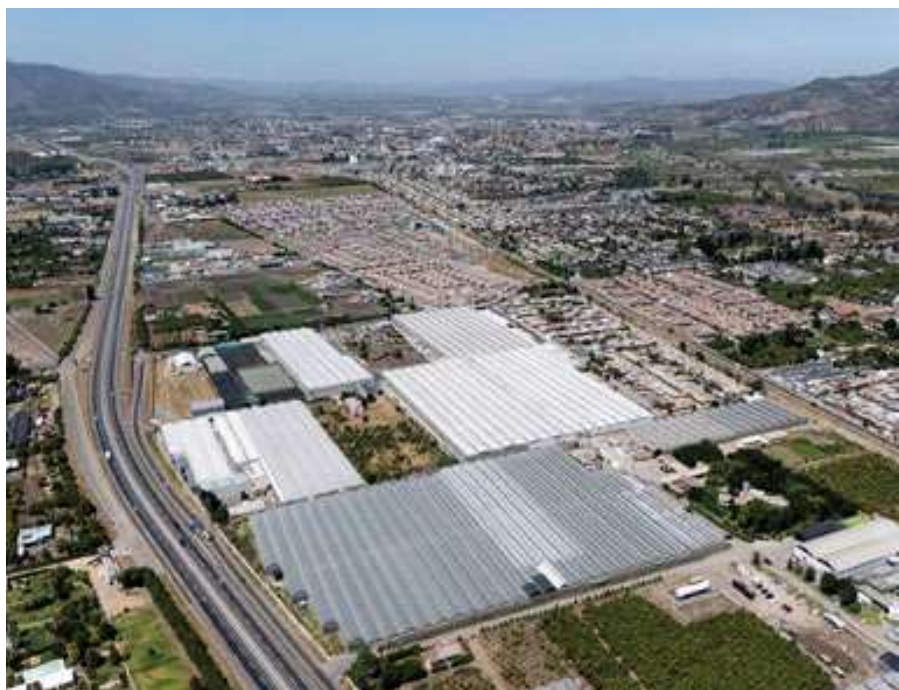
The facility is located 20 km from the ocean, where the climate is temperate.
